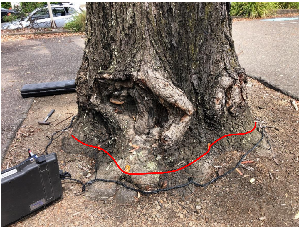
Plate 4: South side of test area. Red line is the approximate location of the test. P. Vezgoff.
